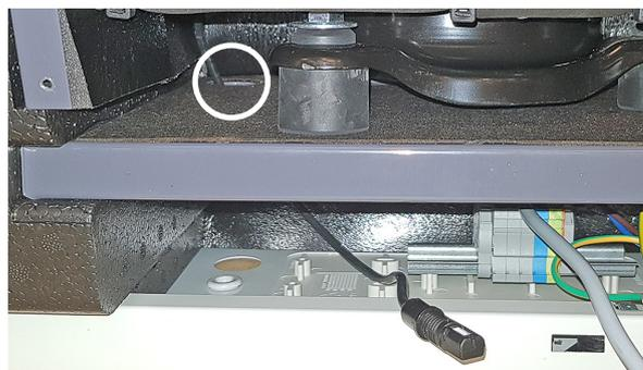
3. Find the compressor compartment cover with the pre-mounted bracket for the humidity sensor.
